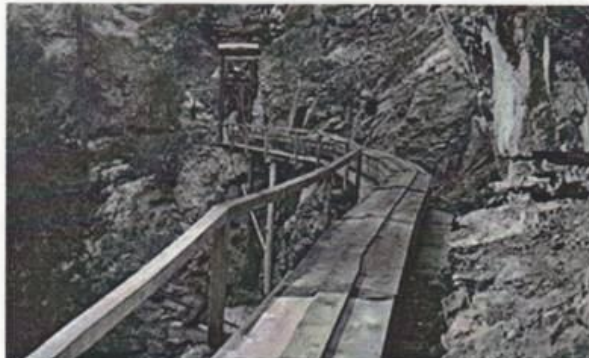
The irrigation system that fed water to the people at Fintry from the falls up above.
