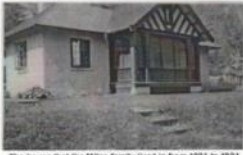
The house that the Milne family lived in from 1921 to 1924 while Mr. Milne worked as the herdsman at Fintry.
