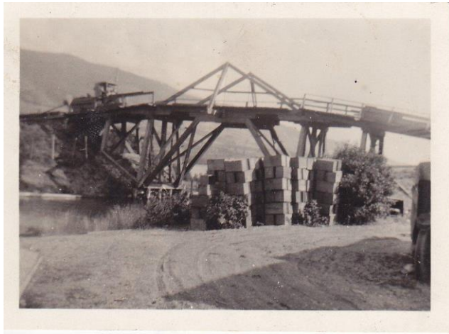
Oyama Canal Bridge – image source Lake Country Museum and Archives, Dorthea Allison Collection.
